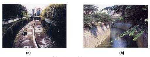
Figure 4: The Condition of Meguro River (a) Before and (b) After the Restoration using Reclaimed Wastewater
